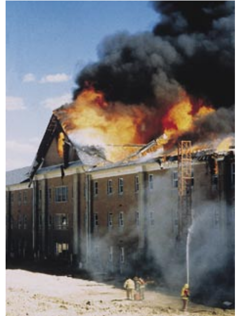
Fanned by high winds, a fire raged in the wood roof framing of this mostly precast concrete structure of the Oaks at Medina continuing-care facility in Medina, Ohio. The fire burned for four hours, leaving some concerned about how extensively the building was damaged and how long it would be before the building could be repaired.
